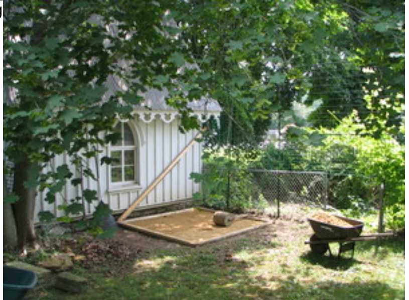
Rough placement of ties before leveling
