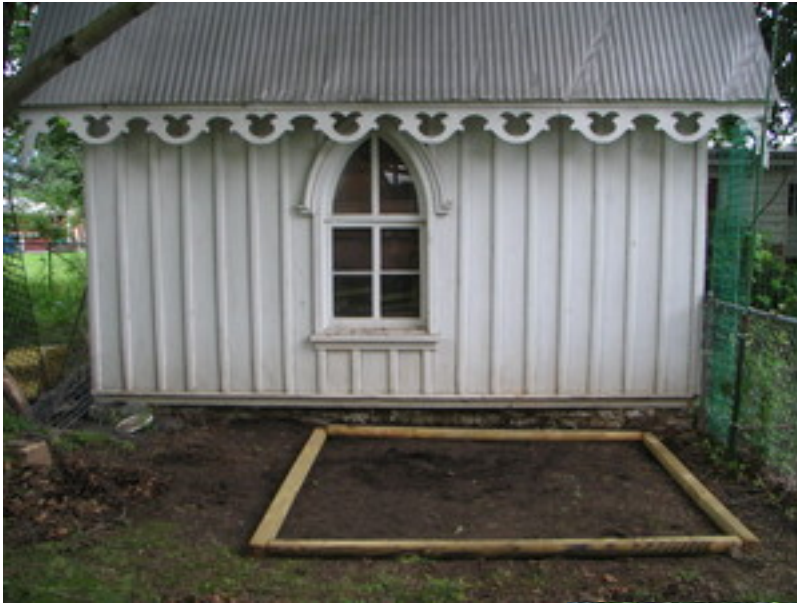
Rough placement of ties before leveling
