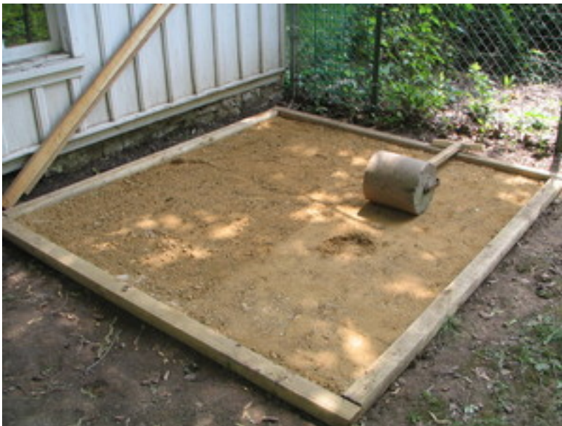
Repaired roller, screet in background; front is compacted
