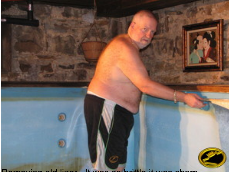
Removing old liner. It was so brittle it was sharp
